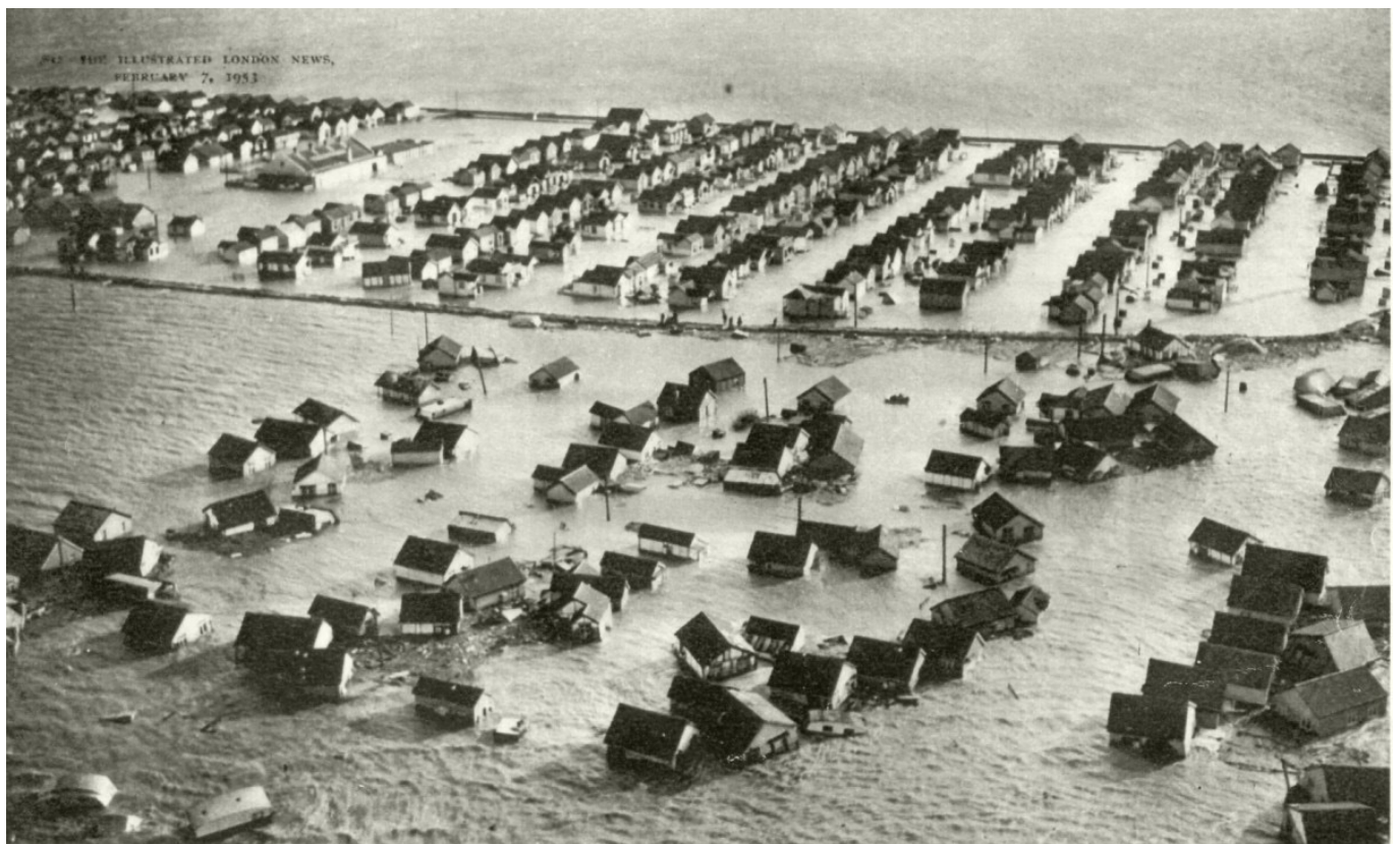
THE ESSEX BUNGALOW TOWN OF JAYWICK, NEAR CLACTON, AFTER THE SEA HAD SWEEPED OVER IT : 600 PEOPLE HAD TO TAKE REFUGE ON ROOFS AND SUN BALCONIES UNTIL THEY WERE RESCUED BY SMALL BOATS, AFTER THE FLOOD-WATER HAD SWIRLED INTO THEIR HOUSES ; AND THIRTY-FOUR WERE ON FEB. 2 REPORTED DEAD.
