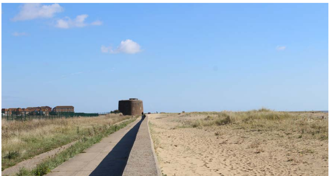
Fig. 7. View looking east from Seawick towards Jaywick Sands and the Martello Tower
