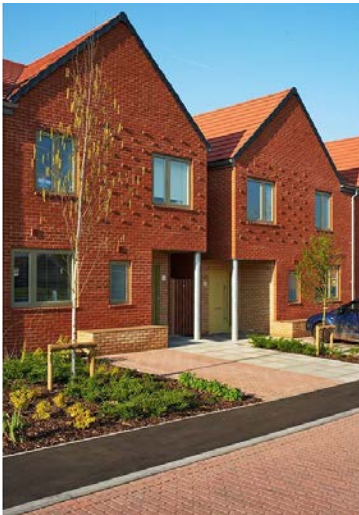
Fig. 59. Use of brickwork neatly detailed
